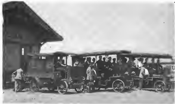
Rapid Cars Loading Passengers at Station for Mudlavia.
